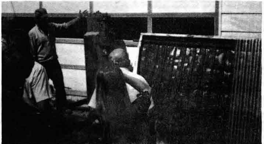
—Martin Kleinschmit describes to farm visitors his solar pre-heat tank and collector under construction at the time.
