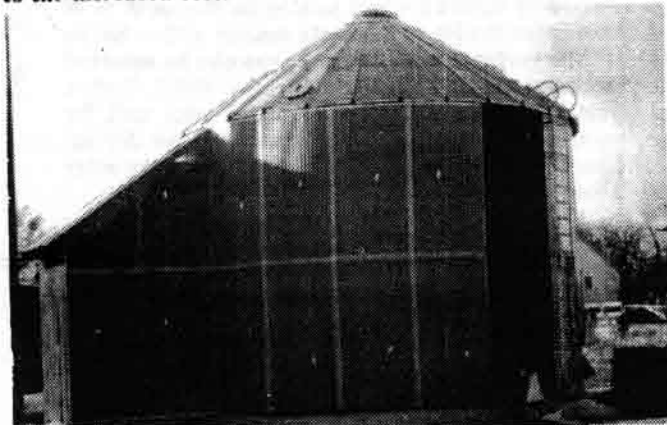
The solar grain dryer on the LaVern Truby farm incorporates a fiberglass cover over the corrugated black metal collector plate shown on the north and right side.
