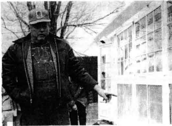
—Earl Fish points out the used storm windows used for the south glazing of the greenhouse. The lower windows were made from screen frames and flat fiberglass.
