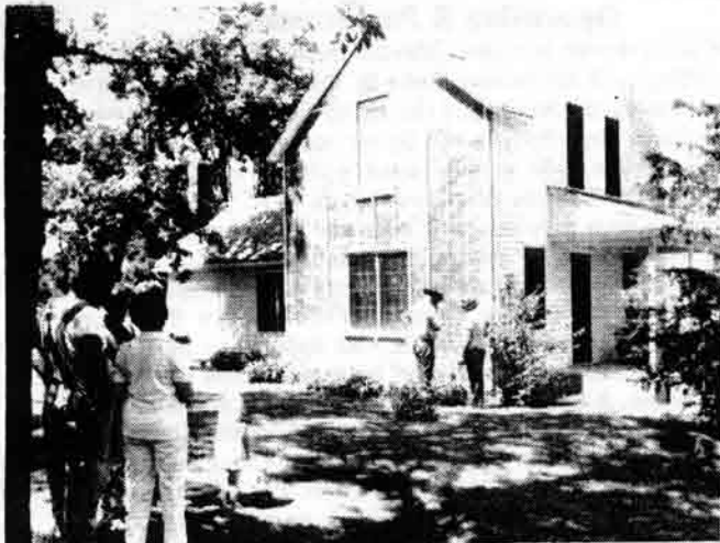
— The vertical wall collector used at the Ken & Jan Stark home. It covers 220 sq. ft. and is used to provide solar heat to the home.
