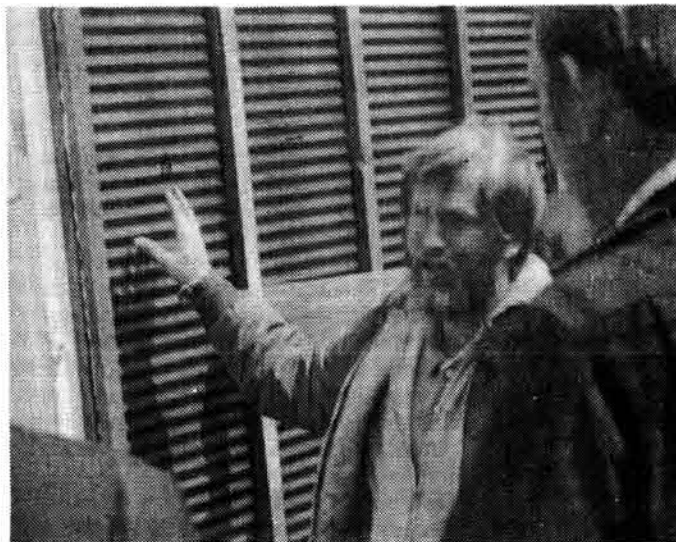
—Ken Stark explains the construction materials used in the vertical wall collector to farm visitors. The photo shows the flat black collector plate before fiberglass was mounted over the vertical 1" wood strips shown. A dead air space exists between the collector plate and the fiberglass cover, with air flow behind the collector plate.
