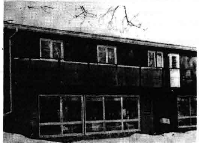
— The vertical wall solar collector on the Paul and Wilma Phelps home is shown on the upper floor. It is 4 ft. x 30 ft. in size and uses a "straight run" air flow pattern which has proved to be the most effective design of collectors used by Energy Project cooperators.
